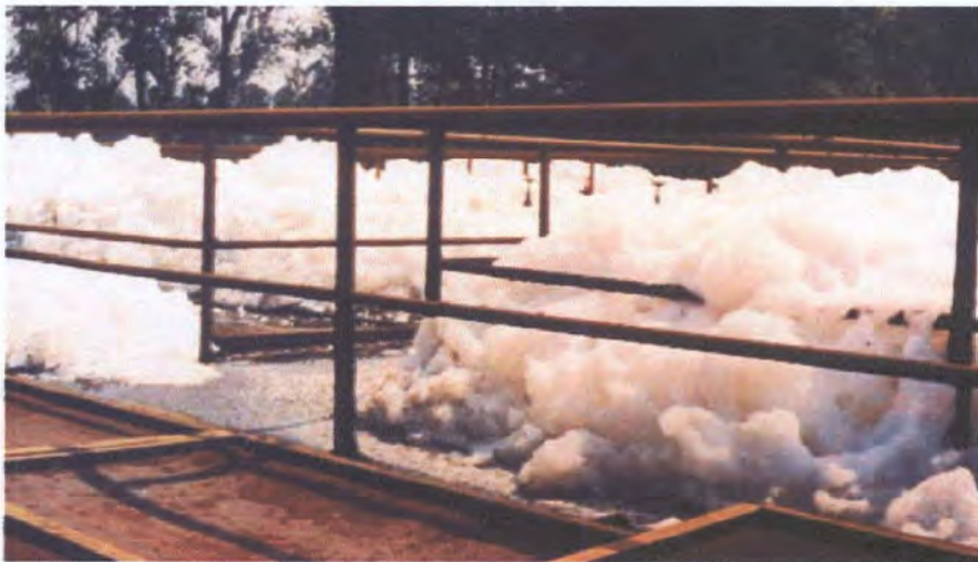
Fig. 2: Foam in a sewage plant
