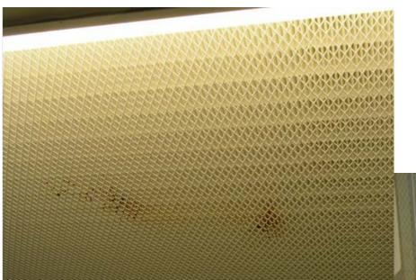
The HEPA filter located immediately above the ISO 5 hood was observed to have stains on the filter surface.
