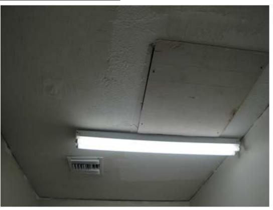
Ceiling above laminar hood which was located in an unclassified room without HEPA filtered air.
