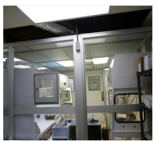
Ceiling above the ISO 6 cleanroom with exposed insulation
