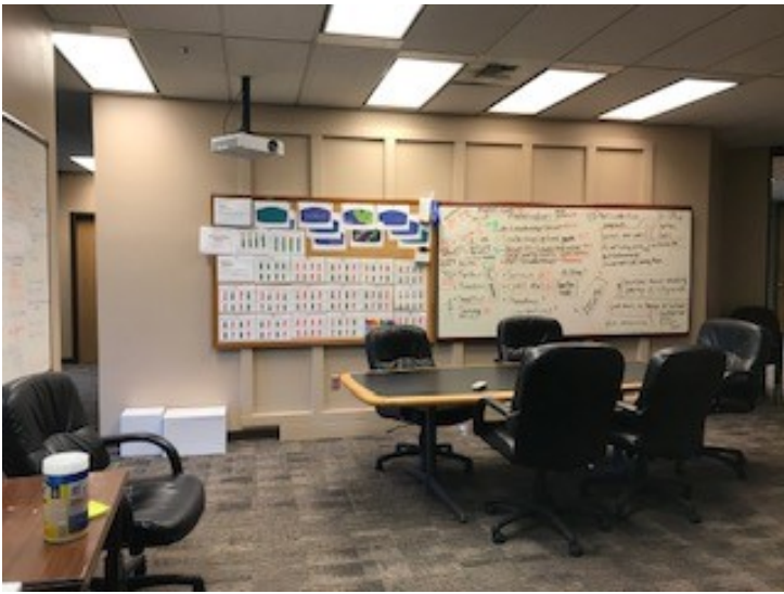
#5 - Removal of entire areas of two offices and doorway, frame/door. SRHD to retain doors/frames. This will be the new area for the cubicles.
