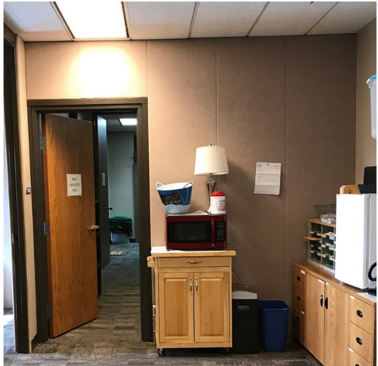
# 2 - Remove wall, doorway to create a hallway. SRHD to retain frames/doors
