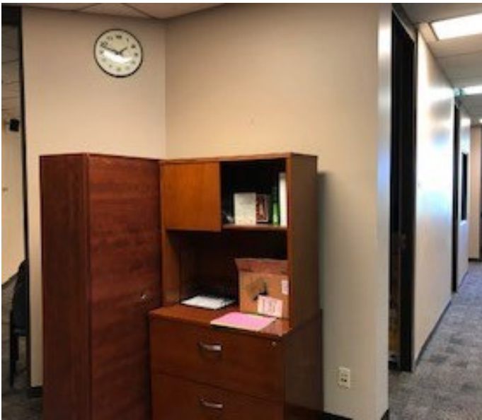
#5 - Removal of this wall, doorway, and both offices
